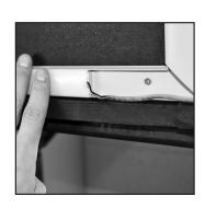
2. Cut WireWay Base to fit full length of cabinet face. Deburr cut edges. Using screws provided, secure Base to bottom of cabinet every 12". (When wiring between adjacent cabinets, drill 1/4" hole through end panels.)
