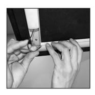
Cut WireWay Cover (or miter piece) to fit exposed Base. Deburr cut WireWay edges. Snap into Base.
